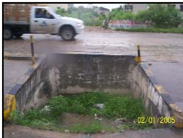
Foto D7.3 Box culvert abs. K00+720
